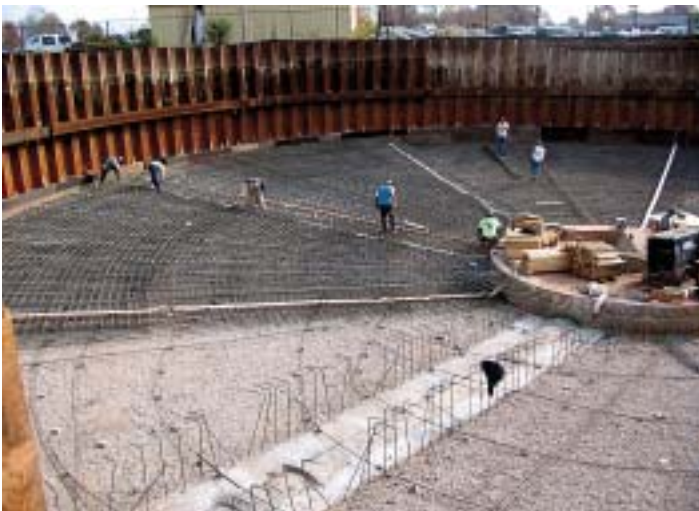
Below right: Rahway Valley Sewer Treatment Project, Rahway, NJ.
