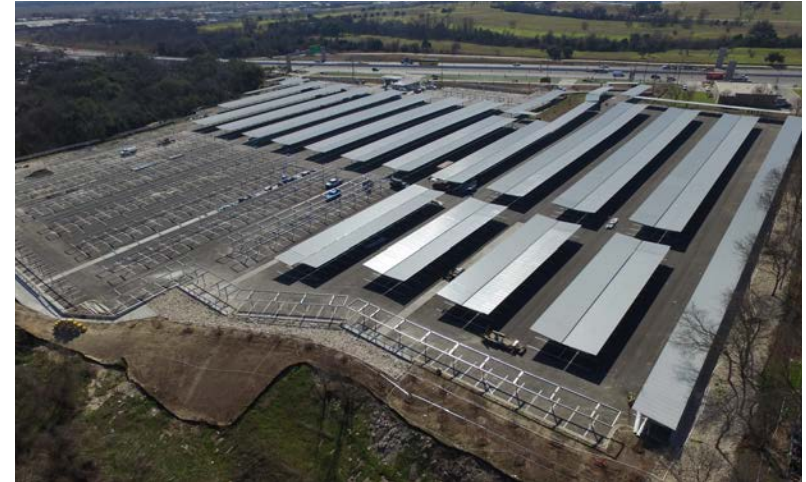
The Parking Spot located at 2935 East State Highway 71, Del Valle, Texas
