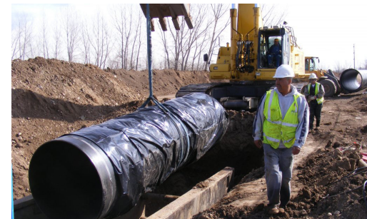
Pipesetting, Greerley, Colorado
