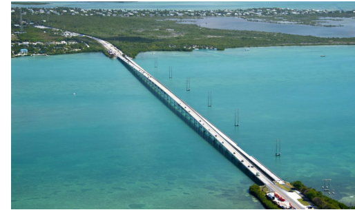
Niles Canal, Key West, Florida
