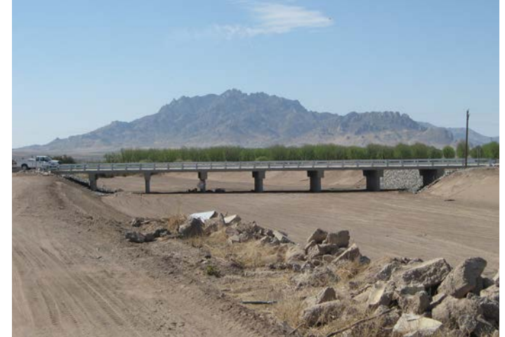
Deming NM Bridge NMDOT Construction
