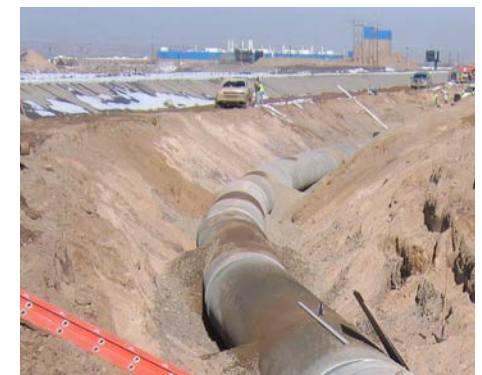
Albuquerque, NM, Raw Water Pipeline ABCWUA Project
