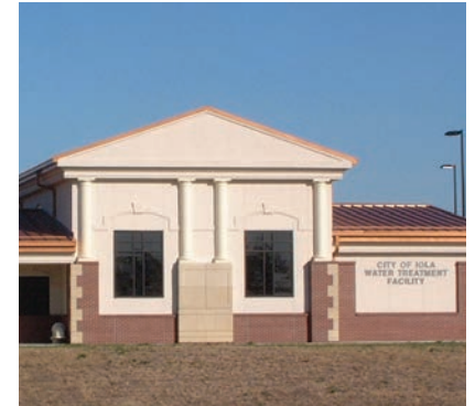
Water Treatment Facility, Iola, Kansas
