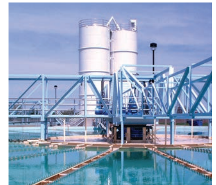
Water Treatment Plant, Topeka, Kansas
